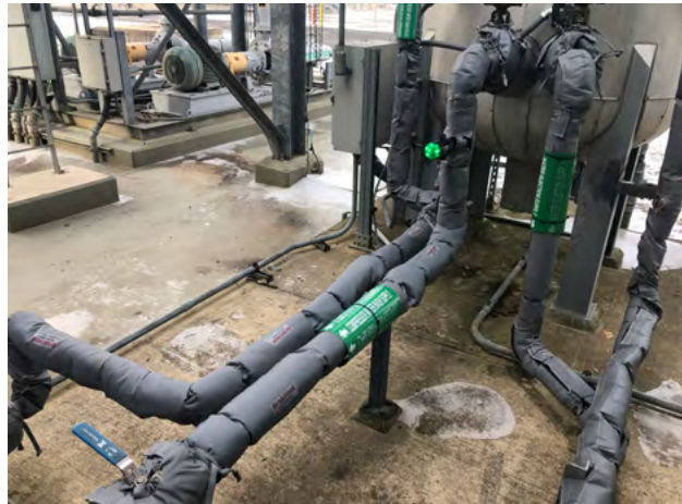
BriskHeat ® Silver-Series removable cloth insulators and self-regulating heating cable
